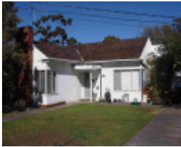
Solomit or Straw House Heritage Precinct ALTONA, Hobsons Bay Heritage Study 2006 - 175 Maidstone Street
