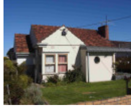
Solomit or Straw House Heritage Precinct ALTONA, Hobsons Bay Heritage Study 2006 - 173 Maidstone Street
