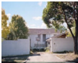
22529 House - 13 Bryson Grove, Lower Templestowe (1)
