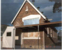
22560 Templestowe Primary School - 1-9 Anderson Street, Templestowe
