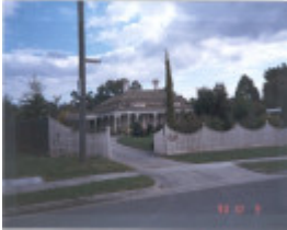
22563 Smith House - 134-136 Atkinson Street, Templestowe
