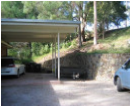
22565 Paringa (carport) - 7 Atkinson Street, Templestowe (4)
