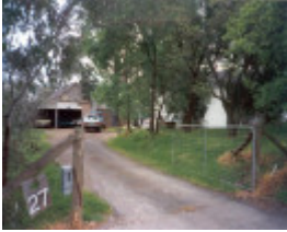
22569 House - 27 Chivers Road, Templestowe (A)
