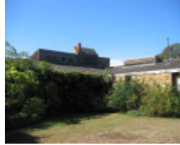
22585 Windrush - 15-17 Homestead Road, Templestowe (3)
