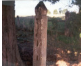
22599 Monckton Gate Posts - 6 Monckton Road, Templestowe (3)
