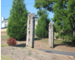
22599 Monckton Gate Posts - 6 Monckton Road, Templestowe
