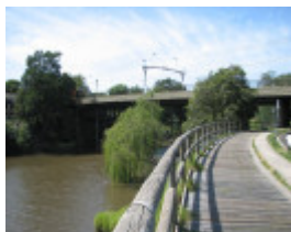
WALLEN ROAD BRIDGE SOHE 2008
