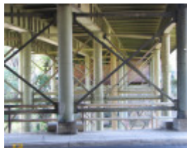
WALLEN ROAD BRIDGE SOHE 2008
