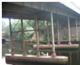
H0380 Wallen road bridge richmond feb07 renee 3
