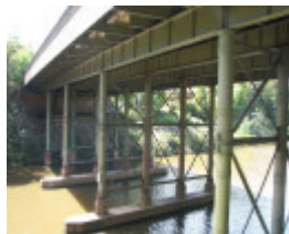
WALLEN ROAD BRIDGE SOHE 2008
