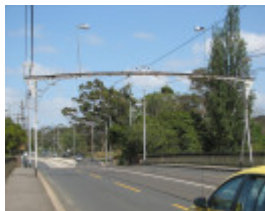
WALLEN ROAD BRIDGE SOHE 2008
