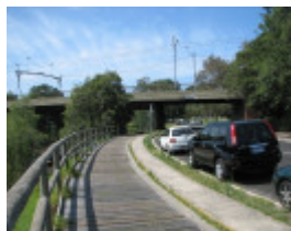
WALLEN ROAD BRIDGE SOHE 2008
