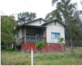
22631 Cottage - 14-20 Brackenbury Street, Warrandyte
