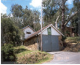
22648 Warrandyte Fire Station (former) - Mitchell Avenue, Warrandyte
