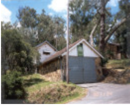
22648 Warrandyte Fire Station (former) - Mitchell Avenue, Warrandyte
