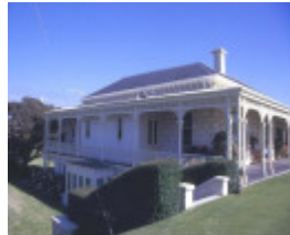
h01899 the anchorage nepean hwy sorrento west view she project 2003
