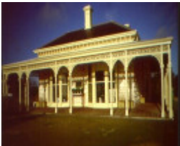
h01899 the anchorage sorrento nepean hwy
