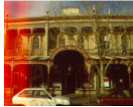
1 holdsworth buildings 380 lygon street h74 july 2000
