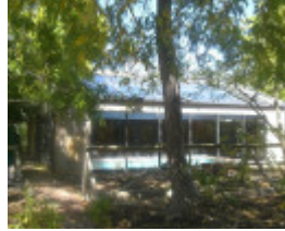
22724 House - 138-140 Brysons Road, Warrandyte South (3)
