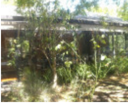
22724 House - 138-140 Brysons Road, Warrandyte South (1)
