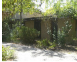
22724 House - 138-140 Brysons Road, Warrandyte South (2)
