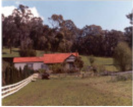
22728 House - 81 Brushy Park Road, Wonga Park
