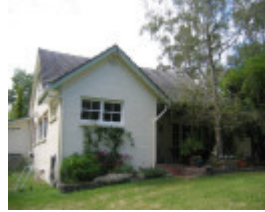
22731 House (rear) - 9 Cecil Street, Wonga Park
