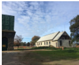
Cocoroc farm hall and Water Tank - June 2020
