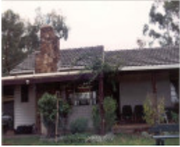
22738 Yarra Brae Cottage - 8 Davis Road, Wonga Park
