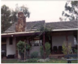
22738 Yarra Brae Cottage - 8 Davis Road, Wonga Park
