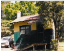
22750 Cottage - 114-116 Jumping Creek Road, Wonga Park
