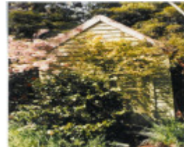
22750 Office - 18-20 Hartley Road, Wonga Park
