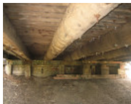
Swan Hill Bridge_Swan Hill_Feb 2008_mz_Round Timber Girders
