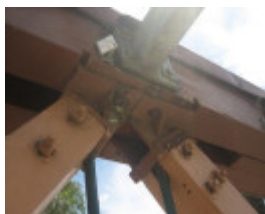
Swan Hill Bridge_Swan Hill_Feb 2008_mz_Truss Connector Detail
