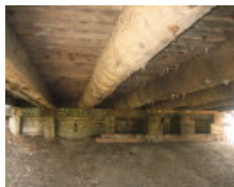
Swan Hill Bridge_Swan Hill_Feb 2008_mz_Round Timber Girders
