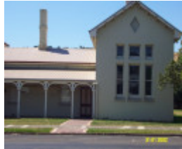
23063 Wannon Shire Offices Coleraine 0428
