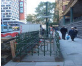
Underground public toilet_Flinders Street_April 2007_view from west
