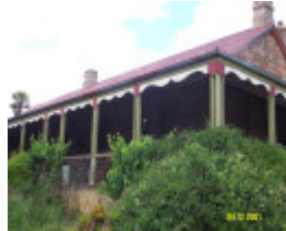
23132 Clunie Homestead front verandah 0272
