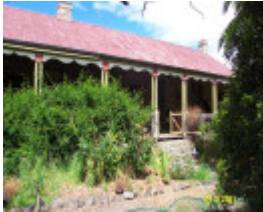
23132 Clunie Homestead front verandah 0270
