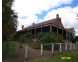
23132 Clunie Homestead front verandah 0271
