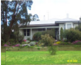
23166 Hospital Former 99 McKebery St Coleraine 1508
