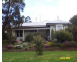
23166 Hospital Former 99 McKebery St Coleraine 1509
