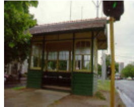
1 tram shelter cnr st kilda rd & dorcas st south melbourne
