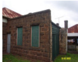
23199 Victoria Hotel Former 100 Bell St Penshurst 1523
