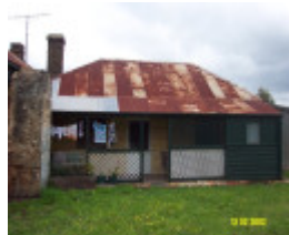
23199 Victoria Hotel Former 100 Bell St Penshurst 1524
