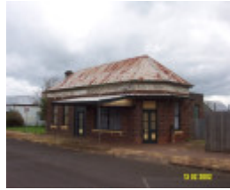
23199 Victoria Hotel Former 100 Bell St Penshurst 1521
