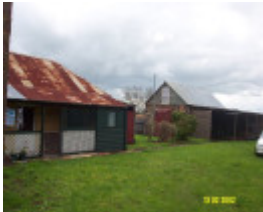
23199 Victoria Hotel Former 100 Bell St Penshurst 1522
