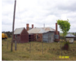
23205 Springwood Homestead Wannon stone cottage 2064
