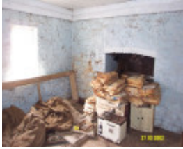
23205 Springwood Homestead Wannon stone cottage interior 2066
