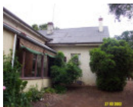
23205 Springwood Homestead Wannon rear 2056
