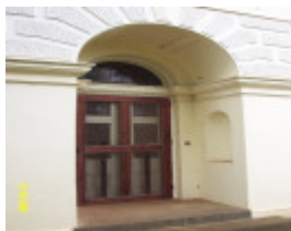
23205 Springwood Homestead Wannon entrance 2049
