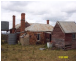
23205 Springwood Homestead Wannon stone cottage rear 2065
