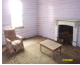
23205 Springwood Homestead Wannon stone cottage interior 2068
