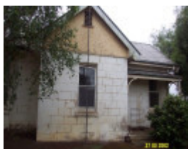
23205 Springwood Homestead Wannon rear cottage 2052
