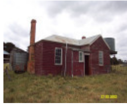
23205 Springwood Homestead Wannon stone cottage extension 2070
