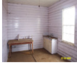
23205 Springwood Homestead Wannon stone cottage interior 2069
