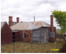
23205 Springwood Homestead Wannon stone cottage 2063
