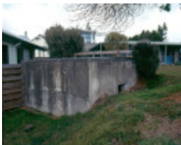
h01090 fort franklin portsea bunker 01 0903 mz
