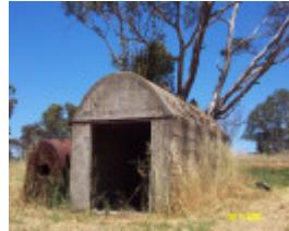
23254 Timber Kiln and Boiler Balmoral 2096
