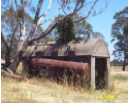
23254 Timber Kiln and Boiler Balmoral 2095
