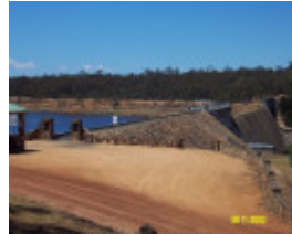
23255 Rocklands Reservoir dam wall 2083
