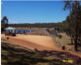
23255 Rocklands Reservoir dam wall 2082
