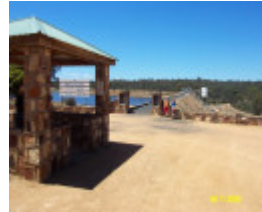
23255 Rocklands Reservoir dam wall 2084
