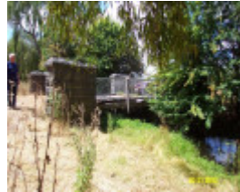
23277 Bluestone Mill Bridge Byaduk 0388
