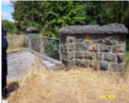
23277 Bluestone Mill Bridge Byaduk 0387
