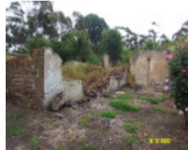
23280 General Store ruins Byaduk 2296
