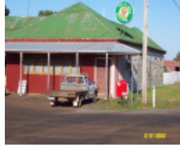
23295 Junction Hotel Branxholme 0470
