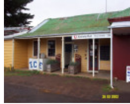
23295 Junction Hotel Branxholme 0562
