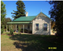
23304 Brae Park Branxholme north side 0724
