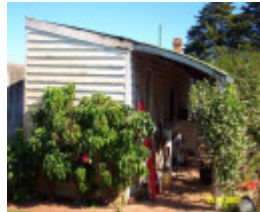
23304 Brae Park Branxholme shed 0722
