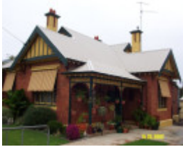
23332 Police Residence Martin St Penshurst 1006
