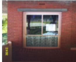
23333 Free Press Building 90 Bell St Penshurst 0801
