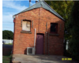
23333 Free Press Building 90 Bell St Penshurst 0802
