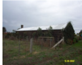
23350 Bluestone Stable and Barn Kennedy Cox Penshurst 0975
