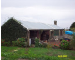
23350 Bluestone Stable and Barn Kennedy Cox Penshurst 0974
