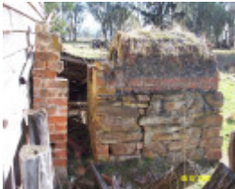
23404 Ruined House Mirranatwa oven 1139
