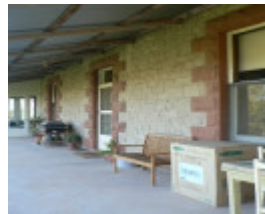
23406 Barra Head Homestead Mirranatwa front verandah 865
