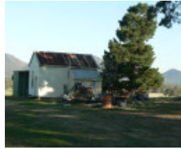
23406 Barra Head Homestead Mirranatwa rear building 861
