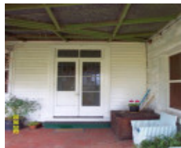
23419 Lovatdale Glenthompson detail of verandah 1234
