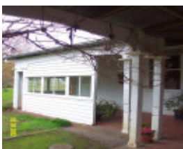
23419 Lovatdale Glenthompson detail of verandah 1235
