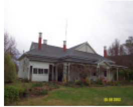
23419 Lovatdale Glenthompson facade 1233
