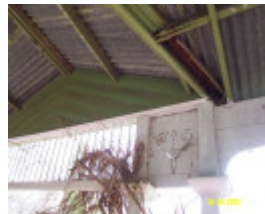
23419 Lovatdale Glenthompson detail of verandah 1236
