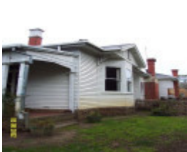
23419 Lovatdale Glenthompson west elevation 1229
