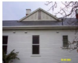
23419 Lovatdale Glenthompson west elevation 1238
