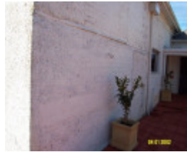
23423 Kinvonvie Yulecart detail of early wall 1312
