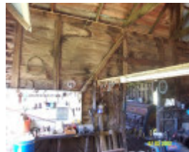
23426 Woodhouse stables slab wall 1741
