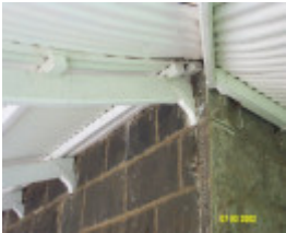
23426 Woodhouse verandah detail 1733
