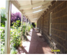
23426 Woodhouse front verandah 1732
