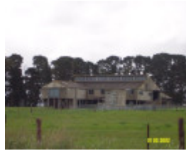
23441 Torbank Woolshed Tobermory Rd Penshurst 1715
