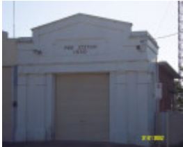
23449 Fire Station Coleraine 0462
