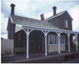
Source: Victorian Heritage Register. Taken 1984.
