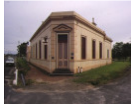
1 bank of victoria bay street port albert front view
