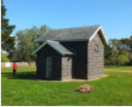
Former Bannockburn Lock Up
