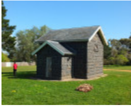
Former Bannockburn Lock Up
