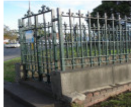
Underground toilet_West Melbourne_May 2007_railing detail
