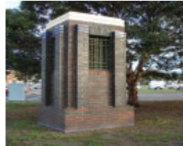
Underground toilet_West Melbourne_May 2007_brick ventilator
