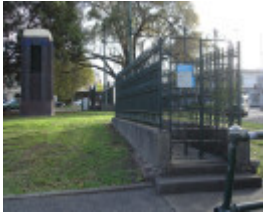
Underground toilet_West Melbourne_May 2007_general view
