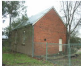
Former Primitive Methodist Church, 2012
