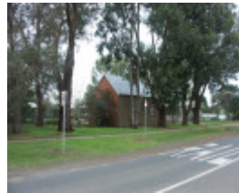
Former Primitive Methodist Church, 2012
