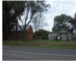
Former Primitive Methodist Church, 2012
