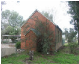
Former Primitive Methodist Church, 2012
