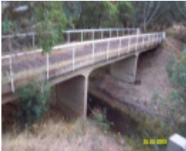
23628 Copy of 4471 Former Wannon Road Bridge Dunkeld
